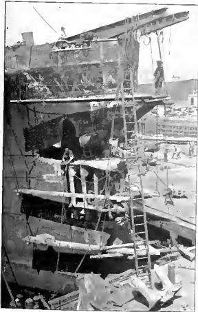
At the left we have the bow of the American tanker Swift Arrow on the dock at the Robins plant of Todd Shipyard Corporation after her collision with the steamship Boston on July 21. At the right is shown the steamship Boston after this collision while undergoing repairs at the Tietjen & Lang plant of the Todd Shipyard Corporation. A feature of this collision was that all the casualties were due to the crushing of passengers in their staterooms. No access was possible to the victims until after the vessel had been towed to port. Had the vessel been equipped with portable oxyacetylene cutting apparatus immediate aid might have been rendered, some lives might have been saved, and certainly much suffering could have been avoided.
